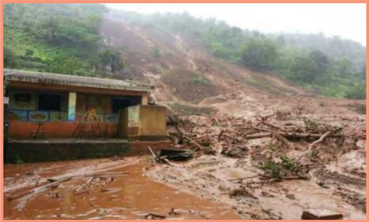
Landslide at Malin Village in Pune District - 2014
