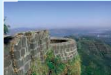
Figure 1.13 : Khadakwasla Dam as seen from Sinhagad
