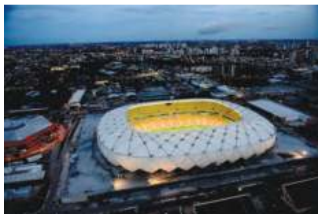
Figure 9.7 : Football Stadium at Manaus
