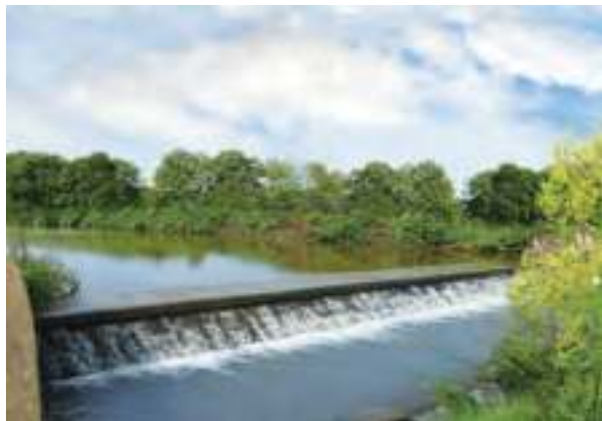
2.3.9 Concrete cement stream check dams
